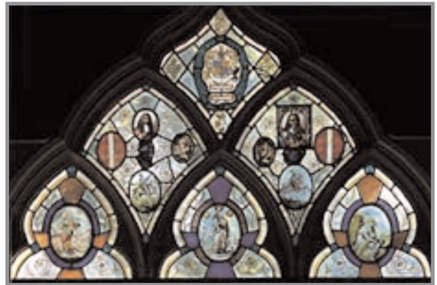
The Library window, July 2006, showing the 1950s layout of Miss Joan Howson, introducing out-of-scale borders in blue and orange around the three lower antique panels and a painted and stained background pattern of roses and foliage, which Dr Peover points out has no historical foundation. Moreover, the quality of glass painting is coarse and inexperienced, clashing with the refined, small-scale style of the antique originals from various centuries. After lengthy consultation with the architects and English Heritage, it was decided to discard the 20th-century backgrounds. ©Paul San Casciani
